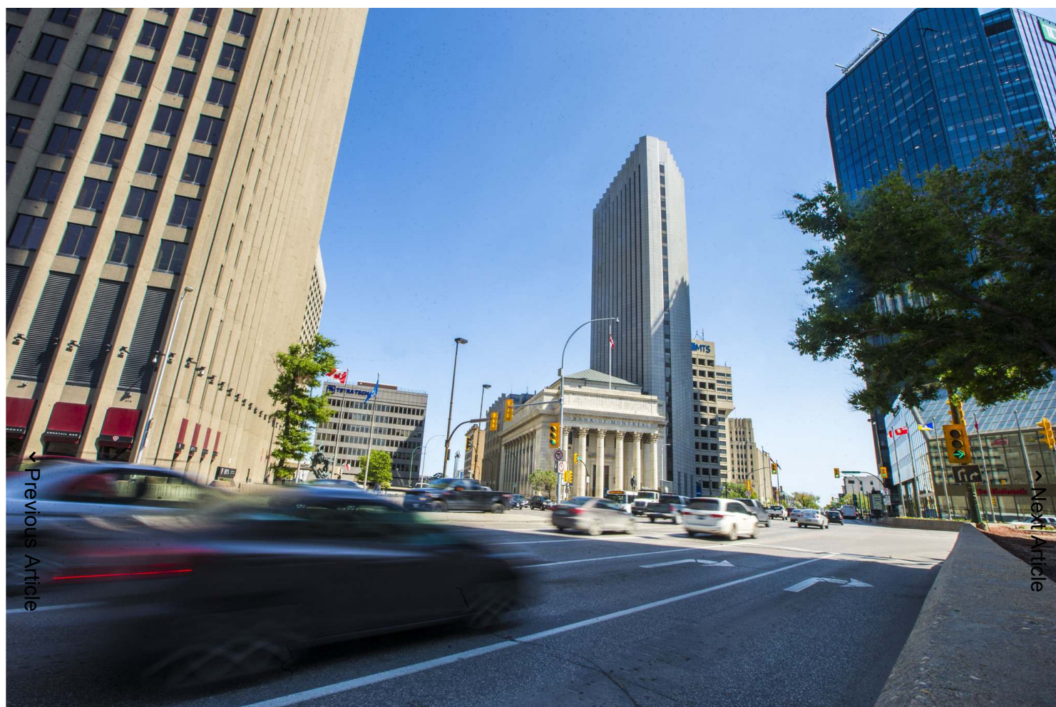
The removal of barriers on Portage Avenue East between the Richardson Plaza and the Bank of Montreal are expected to be part the first phase of construction associated with the intersection re-opening. (Mikaela MacKenzie / Winnipeg Free Press Files) MIKAELA MACKENZIE / WINNIPEG FREE
